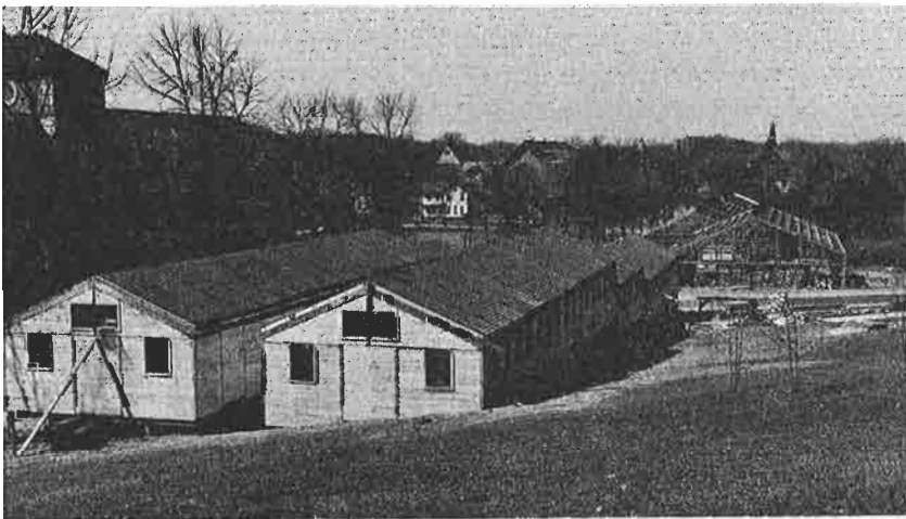
Figure 3.4 Reconstruction of World War II temporary buildings. T-18 in background.
